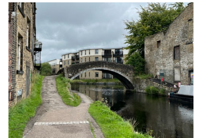
Listed Canal Bridge
